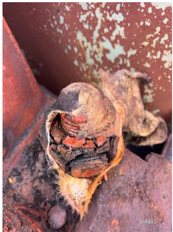
Anchor mooring winch holding down bolt completely wasted and not maintained
