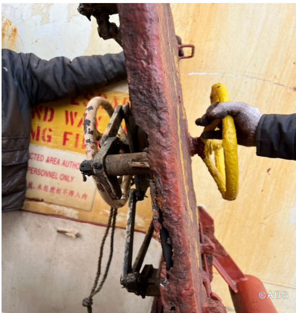
Steering gear room escape unable to close properly and not maintained
